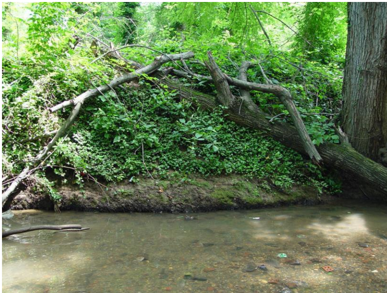
Figure10.Suspended log bank protection.
